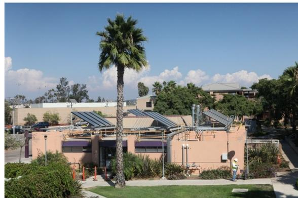
*The Consolidated Bachelors Quarters laundry facilities installed solar panels at Marine Corps Air Station (MCAS) Miramar. The solar panels heat water before it enters the boilers to conserve energy.*
