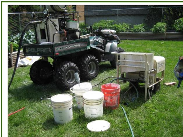
Waupun remediation project now closed. Above, an ATV GeoProbe injecting chemical ORC into soil borings on neighboring WIARNG property at Waupun. Site became contaminated from fuel oil leak on WIARNG property.
