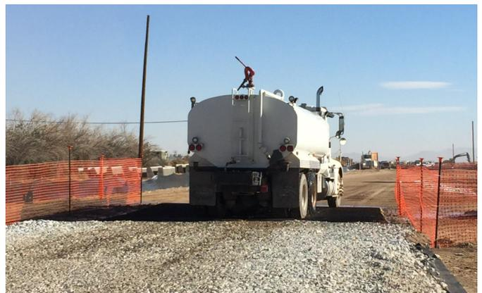
*To mitigate dust, Barstow personnel use watering trucks to spread water over base roadways. A project is now in place to use recycled asphalt, as seen above, that generates less dust so less water is required, therefore increasing resiliency.*
