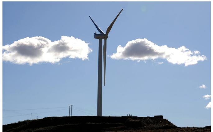
*The Marine Corps Logistics Base Barstow wind turbine generator has been running at 1.0 megawatt for many years. By installing a conditioning monitoring system, the base will be able to run an additional 325 kilowatts. The monitoring system will also aid in preventing very costly equipment failures.*
