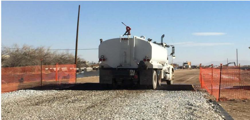
**Dust mitigation is handled by utilizing all-important water resources that watering trucks spread throughout the base. With a project in place to use recycled asphalt, the base will realize increased resiliency and significantly decrease the consumption of water.**
