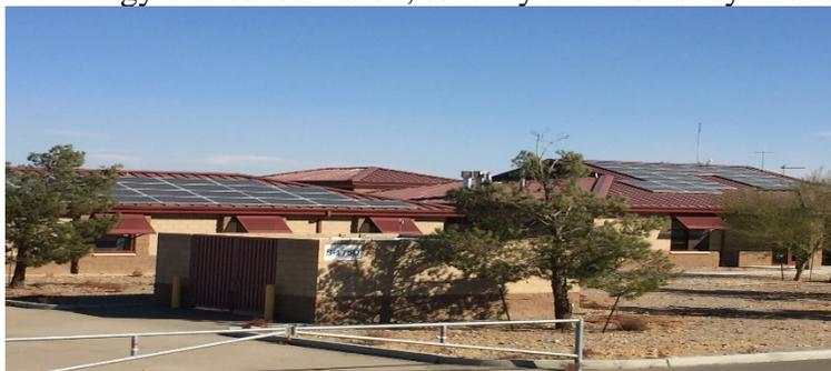
**The Bachelor Enlisted Quarters has 75 kW of solar photovoltaic panels installed on the roof of the building as the nearby carport.**
