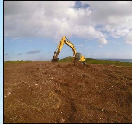
*Figure 4. Remotely-operated equipment cutting and raking vegetation into piles.*
