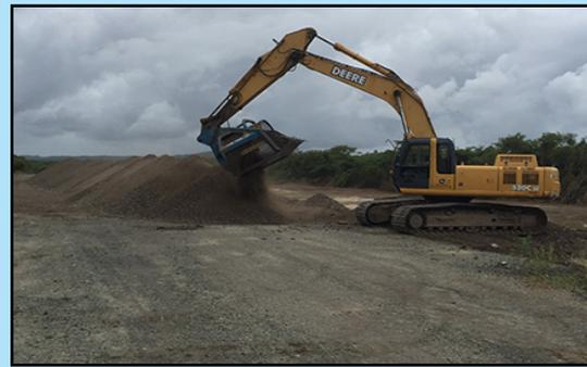
*Figure 6. Preserving virgin material by repurposing runway base course for road maintenance.*
