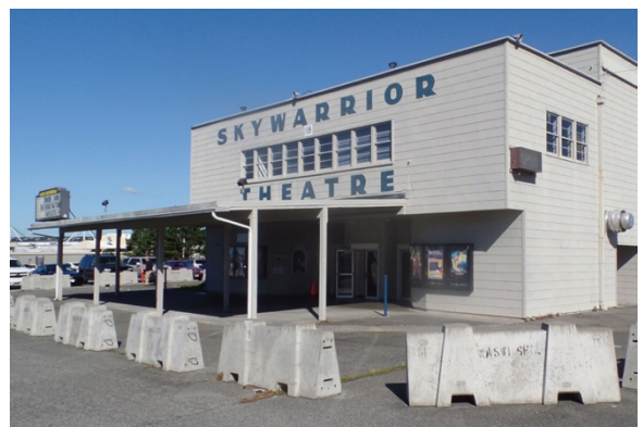
Ault Field, Naval Air Station Whidbey Island. WWII era Skywarrior Theater built in 1942 and in use for the last 75 years. Managed under Skywarrior Theater Preservation and Maintenance Plans. (Photo by the Hardy-Heck-Moore Inc. team. 150921-N-KQ701-001)
