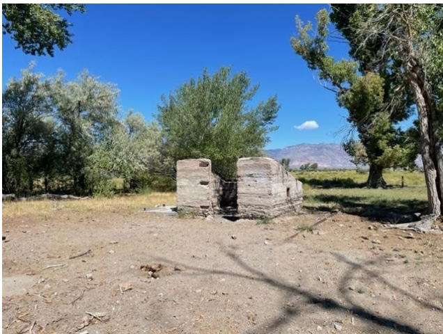
Historic Pump House Located in the Dixie Valley Settlement Area
