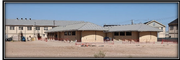
In 2021-22, the CRMT supported the construction of a pair of 3-D printed barracks within the historic view sheds on the Main Cantonment. The new barracks blend into the nearby Cold War-era guided missile labs. These barracks will be the largest 3-D printed buildings in the western hemisphere.
