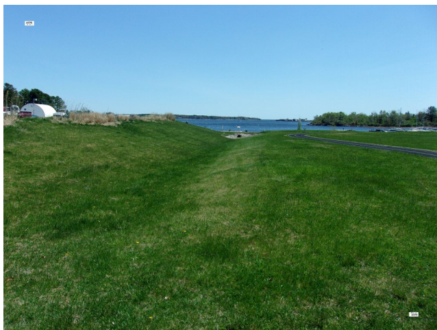
The JILF cap effectively covers hazardous waste within OU 3 while allowing beneficial reuse, including parking and recreational uses. The ER Program is currently partnering with the PNSY CO and XO, NAVFAC PWD-ME PWO and other leadership, and PNSY tenants to evaluate the expansion of much-needed parking facilities on the JILF cap.
