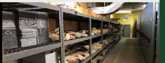
After performing an emergency assessment following the July 2019 earthquakes, the team worked with Public Works personnel and the program management team to execute some accelerated projects, such as replacing wooden shelving with steel reinforced shelving bolted to the wall. The steel shelving is better suited to hold and maintain curation facility artifacts.
