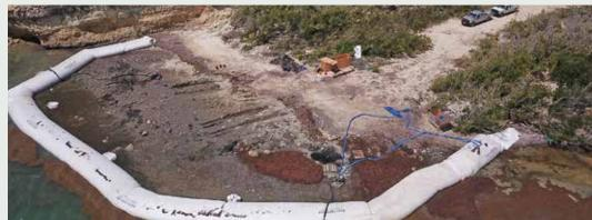
The Vieques Environmental Restoration Team deployed a temporary, water-filled cofferdam to isolate and dry the removal area of an offshore munitions site. This innovative approach allowed UXO technicians to successfully remove munitions without using UXO divers. The cofferdam provided for more effective access by exposing the formerly underwater environment and munitions, thus accelerating the cleanup while increasing the operation's safety.
