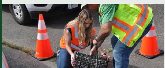
Kelsey Hall and Chris Jorgensen, two environmental engineers within the NAVBASE Kitsap Environmental Division, deploy crates of oyster shells into the stormwater sewer. Oyster shells directly absorb single-constituent metal ion solutions such as zinc and other harmful metals in stormwater, and they are an inexpensive alternative to traditional stormwater treatment methods.
