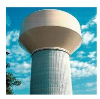
A one million gallon storage tank located on NSA's main campus stores reclaimed water for cooling facilities and infrastructure on NSA's East Campus.
