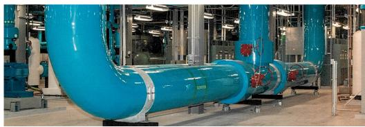
The NSA's chilled water distribution system keeps high performing computer systems cool and functional, allowing critical intelligence community missions across the globe to proceed without impediments. These chilled water pipes are located in the high-performance computing center.
