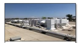
Chemical protective coatings applied to HVAC units reduce the need for maintenance and replacement, and help the equipment operate more efficiently.
