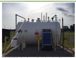
WIARNG Fueling System Upgrade project. Picture depicting upgraded above ground storage tank with new dispenser and leak detection along with system connected to WIARNG Federal network for remote access. Below, new fueling system tank monitoring panel.
