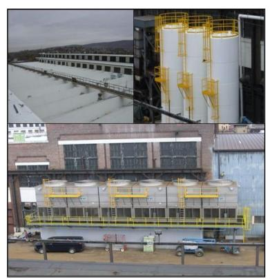
Photo 3: Array of SCAAP Rainwater Collection System. From top left – Rooftop collection basins. Top Right – Collection storage tanks. Bottom – Plant view of collection system in production area.
