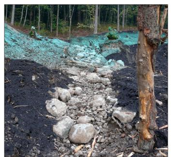
Habitat reconstruction began during the restoration phase. Hydroseeding with native grass species, applying biodegradable geotextile materials, and irrigating with water recycled from the soil treatment system facilitated erosion control and laid the groundwork for this area's future use as hiking and biking trails.
