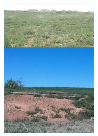
**Landfill 4 After Cover Restoration** Top: The irrigation system running on top of the landfill cover. Bottom: Erosion control measures around the previously eroded areas. Newly emerging grass can also be seen in this photo.
