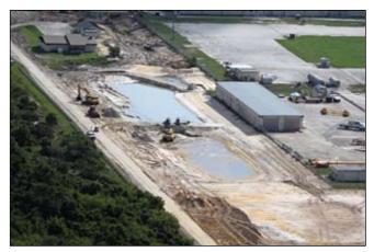
Patrick AFB constructed hydrologic treatment basins to treat contaminated groundwater in a sustainable and innovative way.
