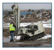
Using the membrane interface probe (MIP) on a direct push rig. This device is able to characterize soil type and screen for the presence of Volatile Organic Compounds in real time. This approach allowed a 12.5 acre site to be characterized in little time and minimized the amount of soil needing removal.
