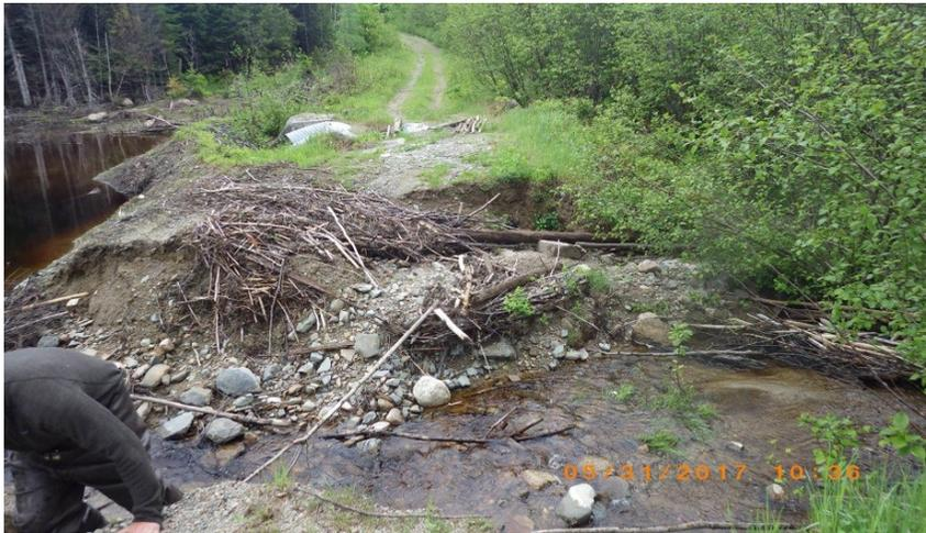
An example of the conditions facing the ENV personnel at WTS. Above, beavers had blocked undersized and “hung” culverts, which caused the road crossing to erode away during spring snow melt. Below, the same site after restoration. A new road has been constructed with storm water turn-outs and an open-bottom box culvert that allows habitat passage and is sized for anticipated future flood flows.
