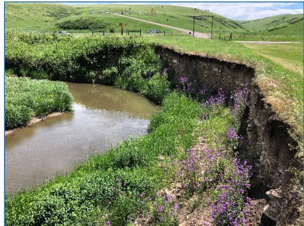
Historic flooding created streambank erosion and encroachment of the mission critical helicopter landing pad. The Team worked with local engineers, construction contractor, and state/local partners to provide innovative solutions for conservation issues and stream bank restoration.
