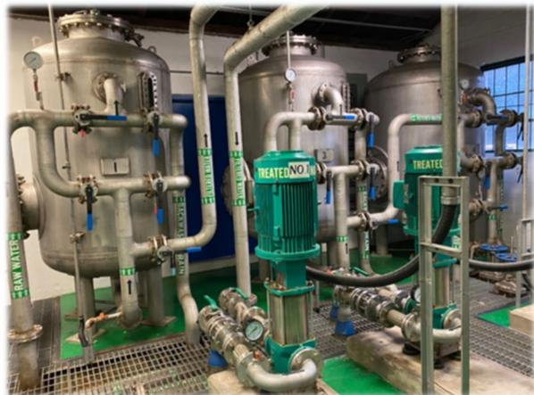
The dual water-filtration system is used to purify groundwater at CFAC.
