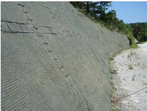
Geotextile installed along slope in 2018, but no sign of germination observed as of May 2019.
