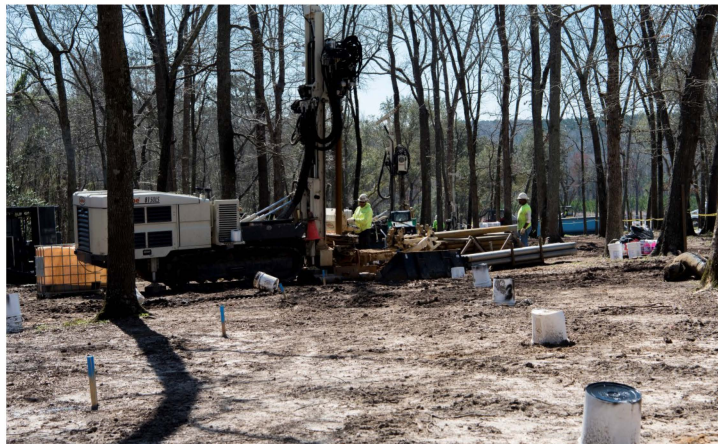
Department of the Air Force environmental restoration contractors use a geoprobe rotary sonic drill rig to drill a small diameter pipe into the ground at Sans Souci Farm in Sumter, SC, March 7, 2019. The pipes are conduits for the precise injection of the BOS 100 product.
