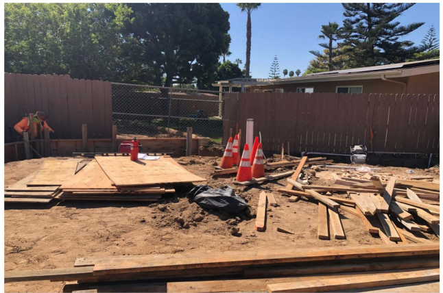
Admiral Hartman Family Housing tot lot construction October 2020.
