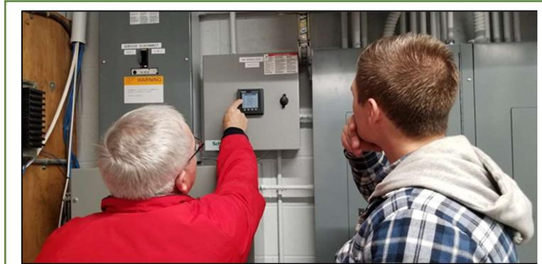
Installation of Army Metering (MDMS) allows FMO Sustainability Team members to monitor building energy usage down to 15-minute intervals for more precise energy management.
