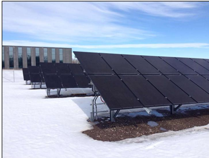
Sustainability Features of the newly constructed Arden Hills Division HQ include a 60 KW solar PV system, expected to meet 2.5% of the expected electrical load, daylighting, solar tube style skylighting, and a ground source heat pump system that will provide for all the heating and cooling needs of the building.
