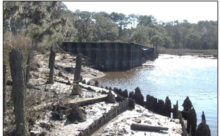
*This tide gate was breached during recent weather events and required repair.*
