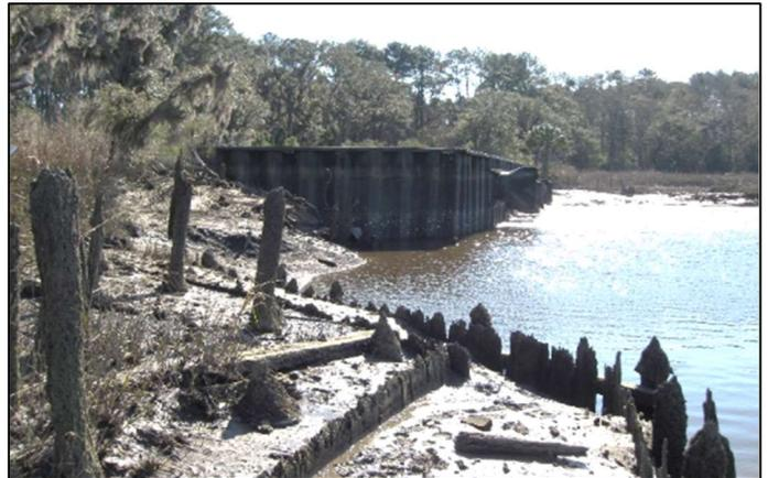
*This tide gate was breached during recent weather events and required repair.*
