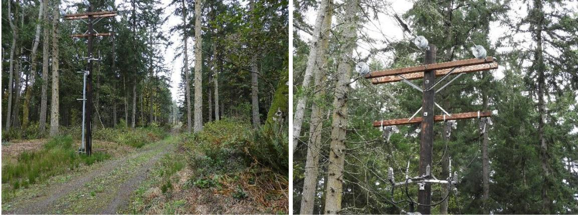
Photos 1 & 2: Shore Power Underground Wetland Buffer and Avian-Safe Phase Conductors
