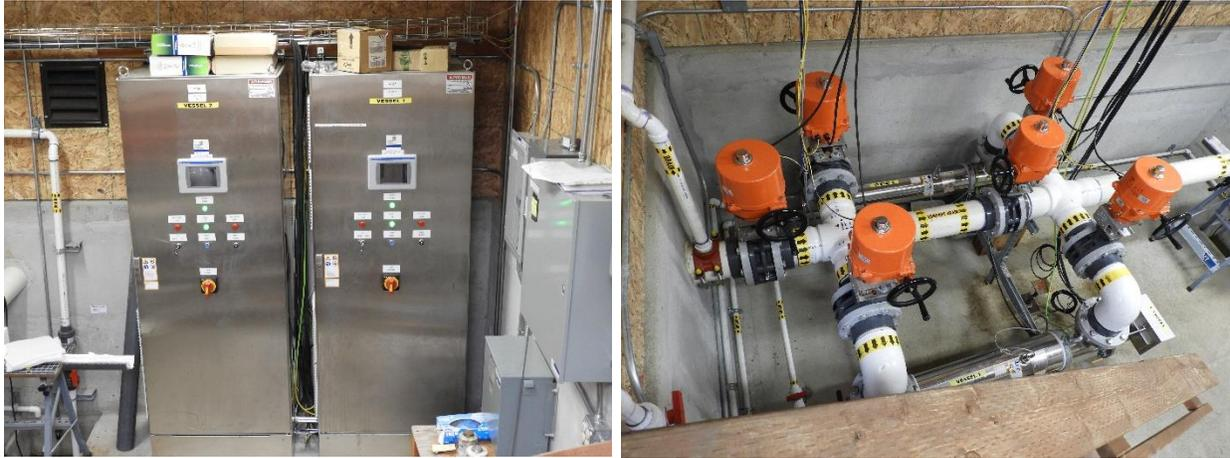
Photos 8 & 9: Ultraviolet Disinfection System at Waste Water Treatment Plant
