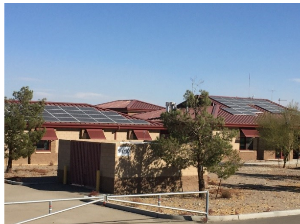
The Bachelor Enlisted Quarters has 75 kW of solar photovoltaic panels installed on the roof of the building and the nearby carport. This increased renewable energy production and reduced energy costs at Barstow.
