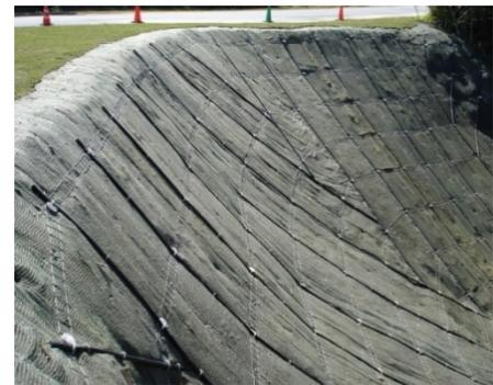
The failed slope near Classroom 1 at the JWTC was effectively stabilized with the use of soil nailing and vegetation matting.
