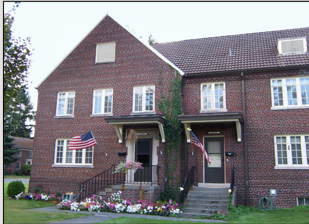
Joint Base Lewis McChord, WA
