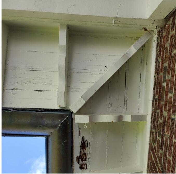
Figure 12: Before image of rotting wood members at JBLM
