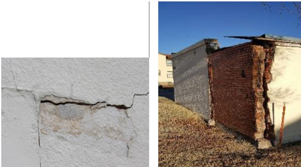
Figure 24: Examples of deterioration of garages in Quanah Parker Square neighborhood, Fort Sill
