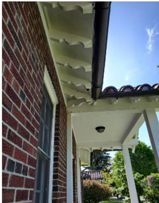
Figure 13: After image of replaced rotting members with in-kind wood
