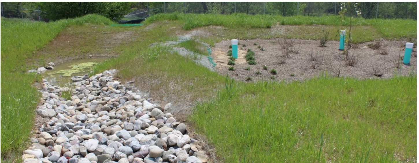
Bioretention project at Fort Detrick, MD. (Photo credit: U.S. Army)
