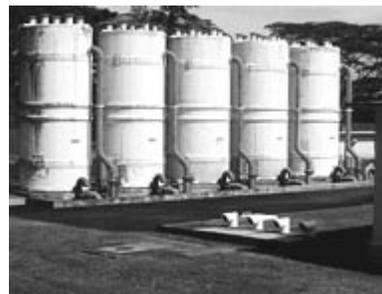
**Schofield Barracks used packed aeration towers for TCE removal.**
