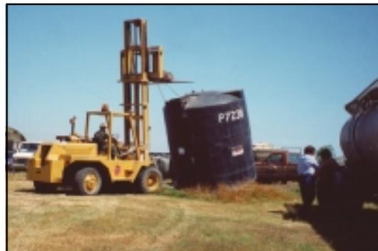
Workers remove an underground storage tank at Los Alamos Armed Forces Reserve Center.
