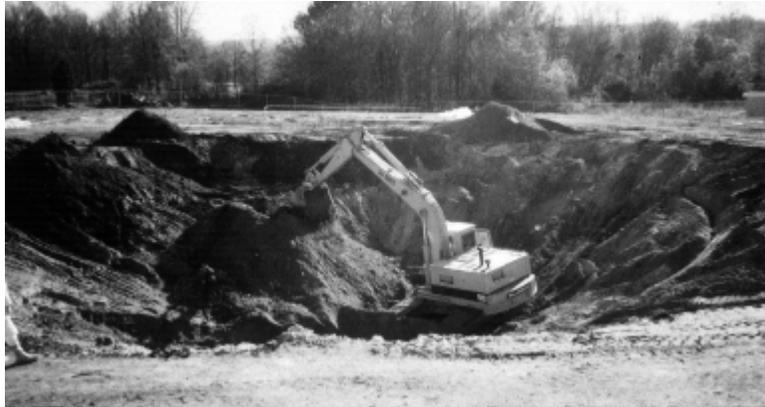
***The U.S. Army Corps of Engineers excavates contaminated soil from the baseball field at the former Raritan Arsenal.***
