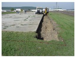
Trenches were dug at the Scotia Depot to remove contaminated soil.
