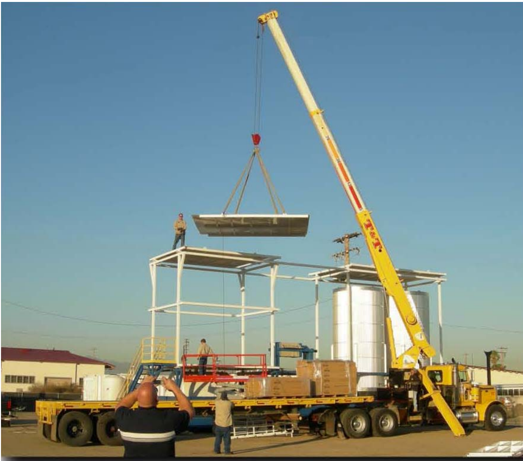
Figure 3. Construction of commercial biodiesel facility at Naval Base Ventura County, CA.
