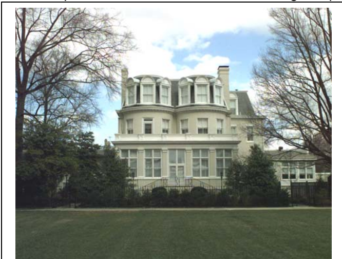
The Home of the Commandants is the last surviving structure of the original establishment of the Marine Barracks in Washington, DC, and has been home to the Commandants of the Marine Corps since 1810. Department of the Navy photo.
