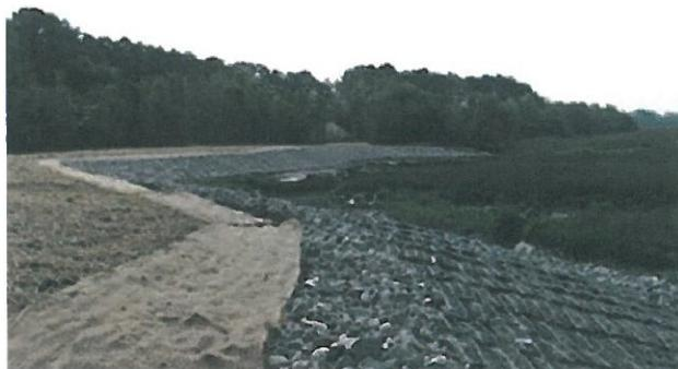
Once in place, the voids within the mattresses are expected to fill with sand and soil from tidal action and natural storm water runoff. Filling of the voids with sediment will encourage the growth of natural rushes and marsh grasses, adding to the mechanical anchors in securing the mattresses in place. The topside of the project was graded and seeded with native grasses.
